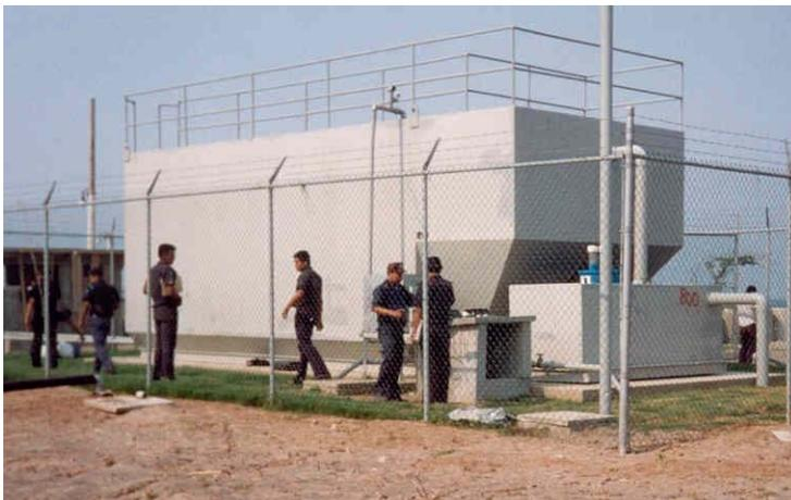
Global’s modular, mobile and deployable Village Systems start with 8’ containers processing 2,500 GPD to 20’ containers processing 15,000 GPD to 40’ containers processing 30,000 GPD.
